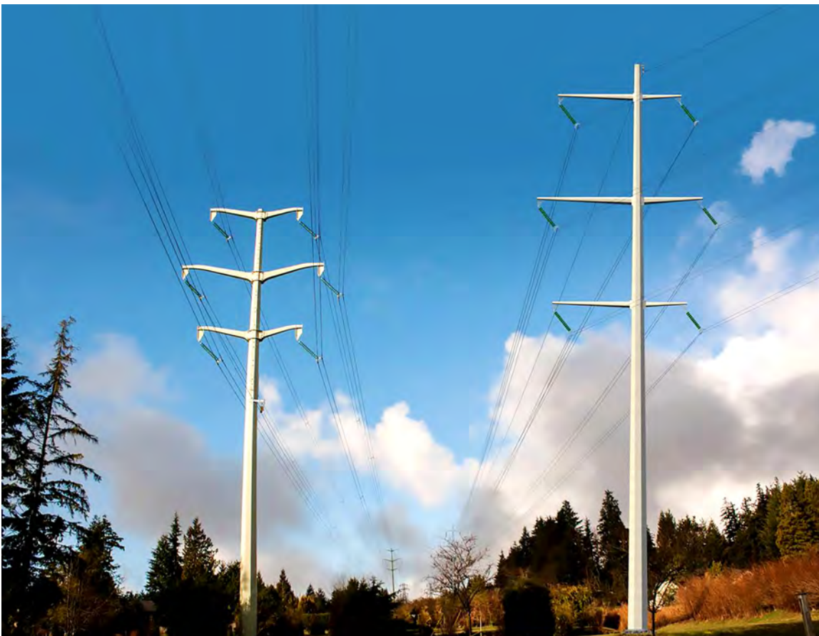
Preliminary rendering showing a new steel monopole replacing a wooden H-frame in Anmore (tower design and placement subject to change). With Alternative 2, there would be 17 fewer poles than existing in the Anmore area.
