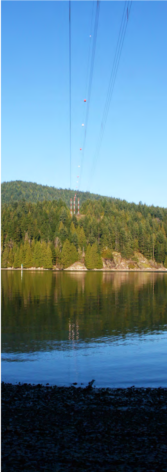
The existing right-of-way crossing Burrard Inlet from Burns Point in Belcarra Regional Park.
