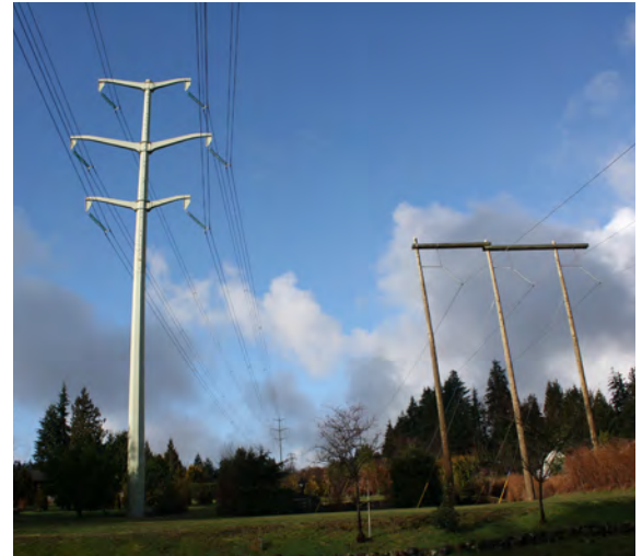
Existing structures (monopole and wooden H-frame) in Anmore.
